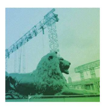
Large format screen support frame featuring Maxitower 52 and RL105A horizontal beams for screens up to 6,000 kg.
