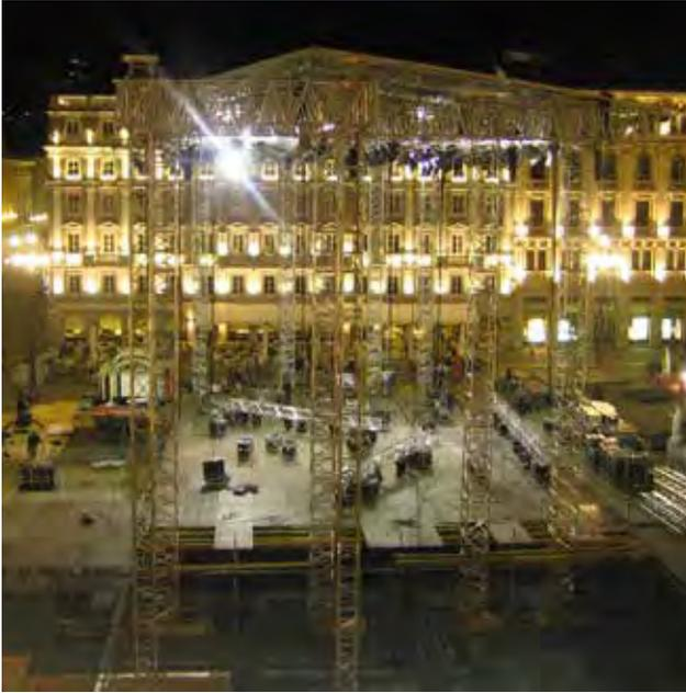
The lifter uses QL76A trusses. It was designed to withstand the stresses that large structures transfer to the ground in their heaviest duty use. It is intended for use together with the LIBERA FL105 system.
