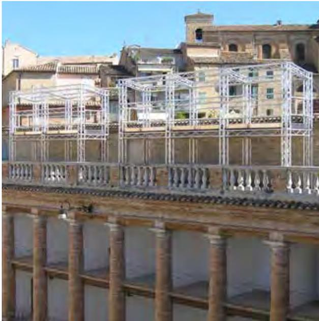
Square section aluminium truss with 25 cm long sides.
