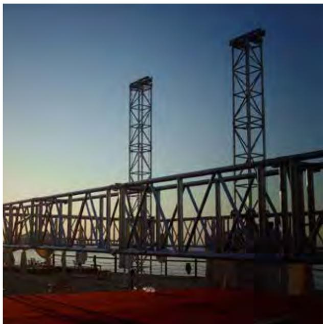
Large format screen support frame for very high load capacity featuring Maxitower 52 and RL105A horizontal beams. The system is truly impressive.
