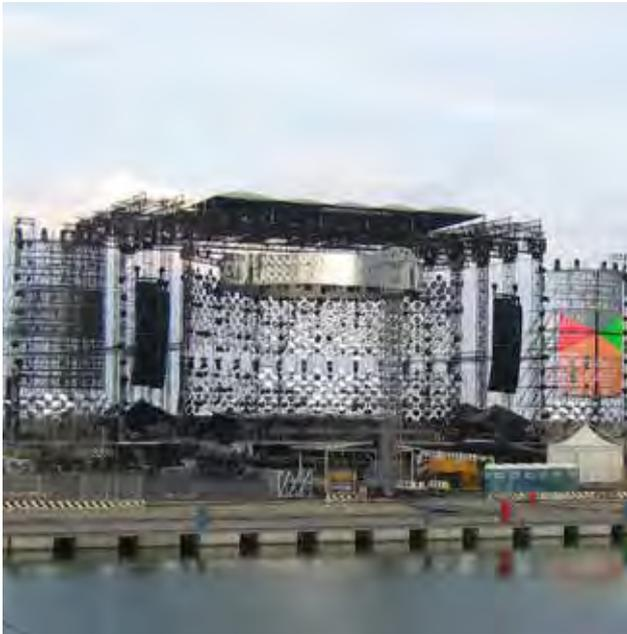
Rectangular section High Load aluminium truss with extraordinary dimensions; it is 84 cm wide, 146 cm high and 500 cm long, and weighs 430 kg. It is made in high-performance aluminium alloy EN AW-7003 T6, among the aluminium series with the best mechanical characteristics. The truss can be used in large installations intended for entertainment, for temporary and semi-permanent structures. At maximum load spans it undergoes virtually no bending.
