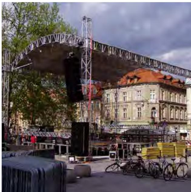
Not just straight: LIBERA can be “bent” and used to create rounded components simply by adding small accessories to normal trusses.
