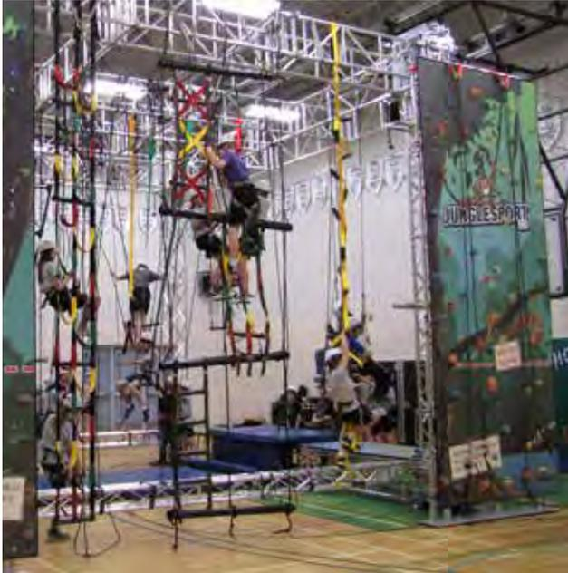
This is the most suitable LIBERA system for fairs and medium-sized installations. This modular grid structure can be used to build single spans of up to 16/18 meters in length with standard centre-to-centre distances (50 cm, 1 and 2 meters).
