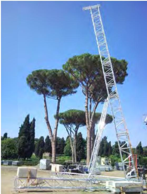
Support tower for for audio systems. Designed in QL52A, this new Flyintower is suitable for 1,400 kg loads and can reach the height of 13 meters, thus ensuring sturdiness and rigidity on relevant heights. It also utilized TX30SA trusses as stabilizing elements and is equipped with fork connections.
