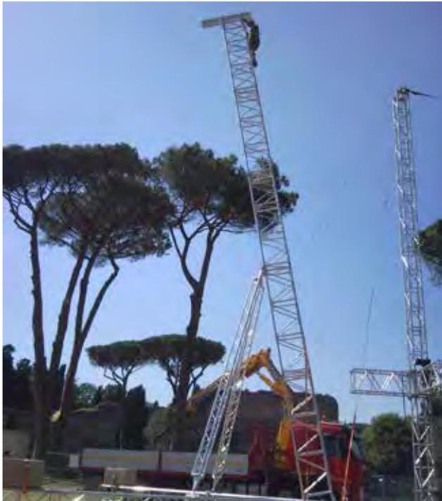
Support tower for for audio systems. Designed in QL40A, this new Flyintower is suitable for 1,600 kg loads and can reach the height of 10 meters, thus ensuring sturdiness and rigidity on relevant heights. It also utilized QH30SA trusses as stabilizing elements and is equipped with fork connections.
