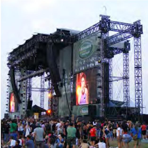
LITEC has deigned the MyT LED screen ground support to fly very heavy screens. The load bearing capacity is 12,000 kg on a maximum height of 20 m.
