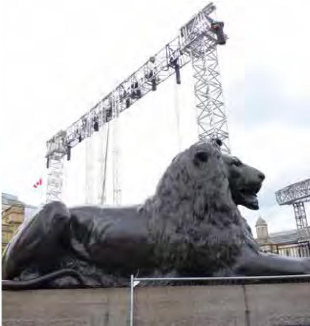
Large format screen support frame featuring Maxitower 52 and RL105A horizontal beams for screens up to 6,000 kg.
