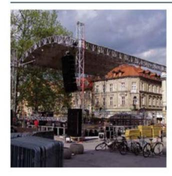
Not just straight: LIBERA can be "bent" and used to create rounded components simply by adding small accessories to normal trusses.
