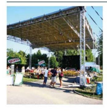
LIBERA is an open structural system. Roof systems in LIBERA 52 consist of Maxitowers and a LIBERA FL52 grid structure. The actual span can reach 16 metres, to which side wings may be added.
