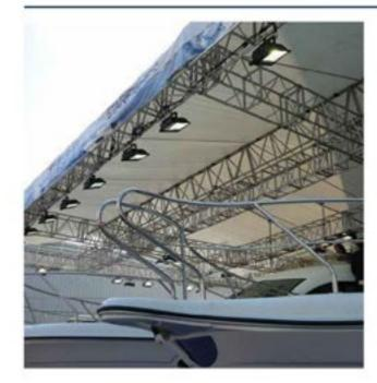
These roof systems are high-performance structures that feature a connection made through steel forks. This line was designed when a high loading capacity is required together with wide spans.
