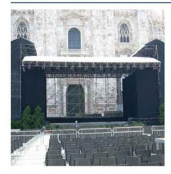
LIBERA is an open structural system. Roof systems in LIBERA 76 consist of Maxitowers and a LIBERA FL76 grid structure.
